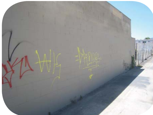
Wall With No Window Facing Creek
