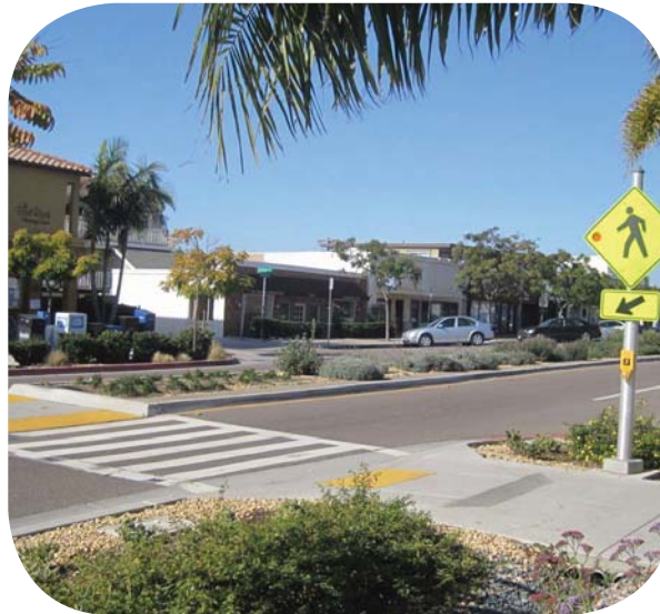
Pedestrian crosswalk with signage, striping, and pedestrian activated LED lights similar to the recently installed crosswalk at 25th Street in Del Mar, CA
