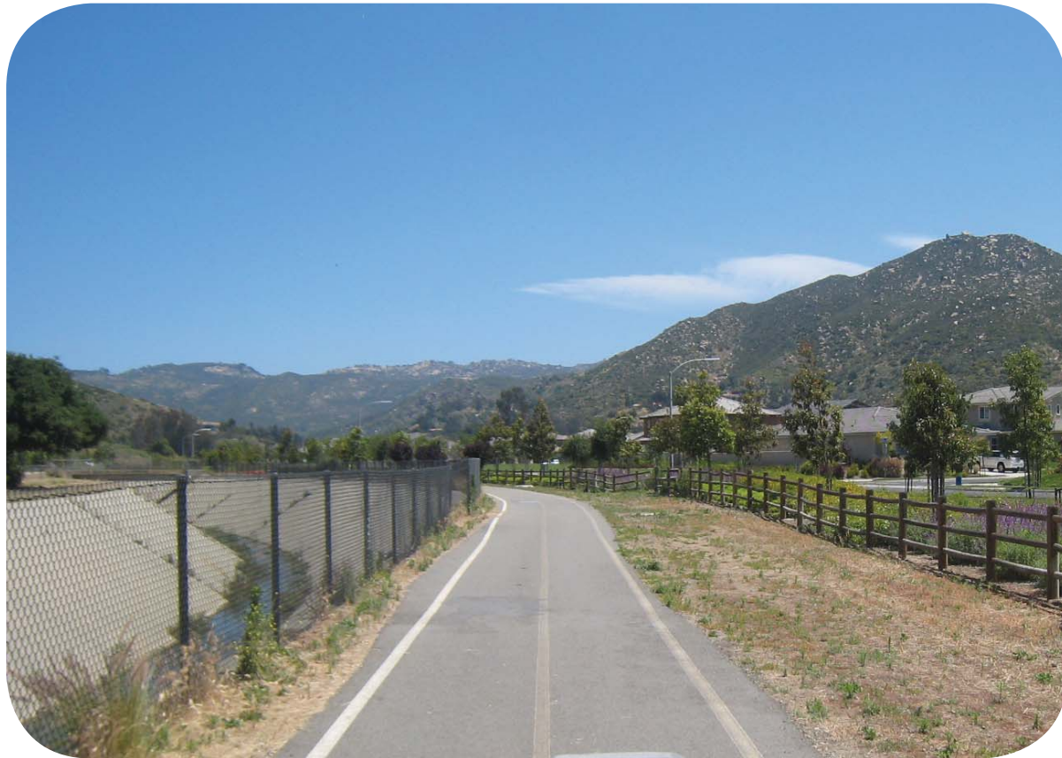
Existing Asphalt Trail
