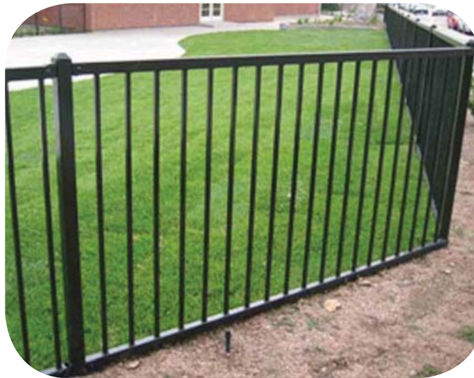
Four Foot High Fencing Proposed at the Top of the Channel to be Black Tubular Steel or Black Metal Wire Fencing with Top Rail
