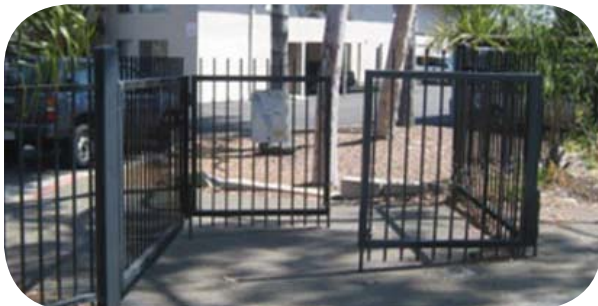
Existing Black Metal Fence near Date Street
