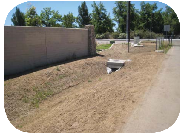
Typical Drainage Swale
