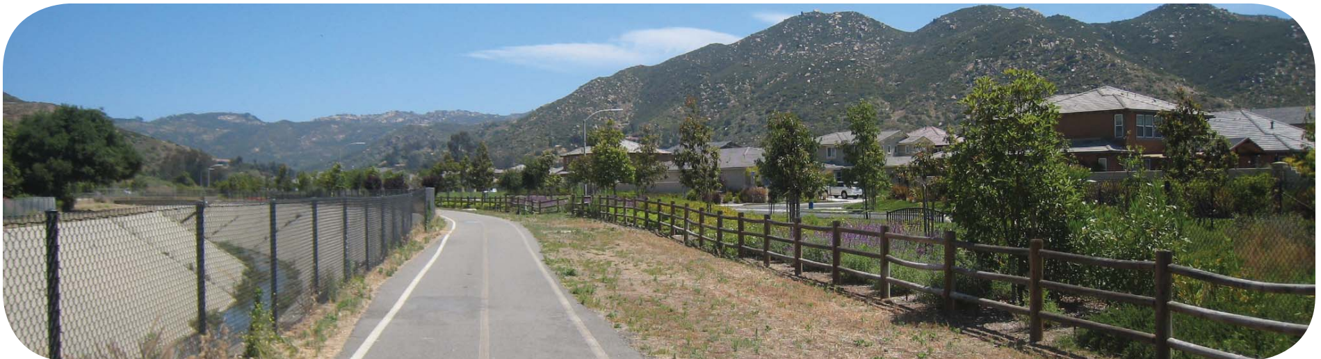
Existing Asphalt Trail
