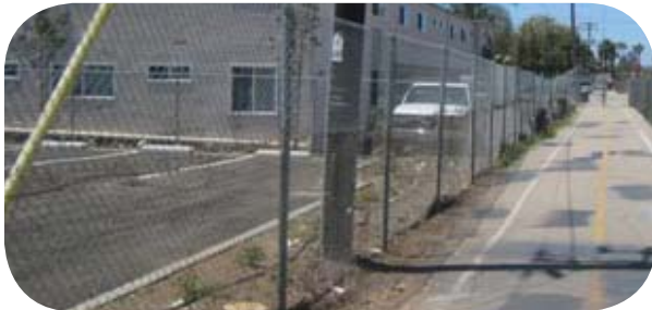
Typical Chain Link Fence along the Trail
