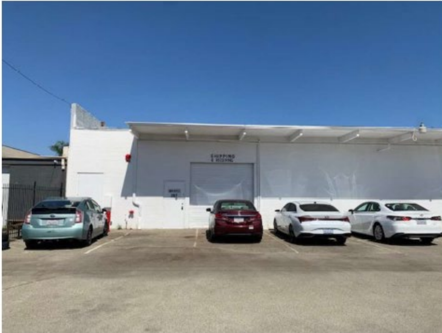
SOUTH SIDE – BACK ENTRANCE / ROLL UP DOOR (TO BE REMOVED AND AN EXTERIOR STOREFRONT WINDOW TO BE PROVIDED INSIDE OPENING)
