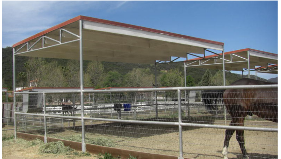
Pipe Rail Corrals with Shade Structure
