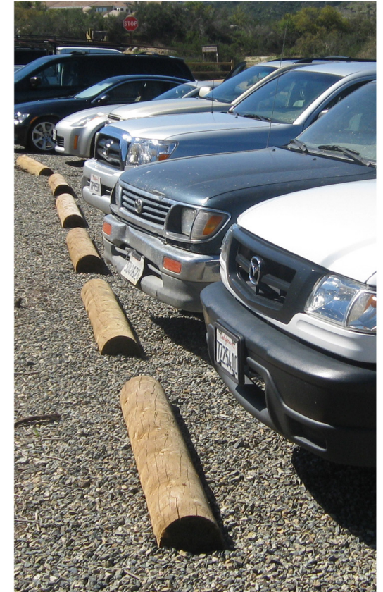
Figure 65: Parking Lot Tire Stops
